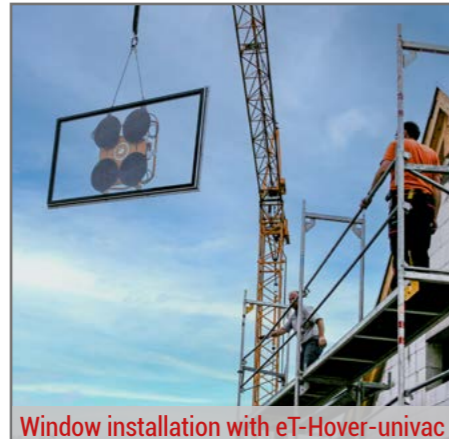
Window installation with eT-Hover-univac
